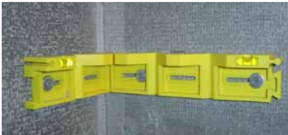
3. Hold first section to mark and secure one end of **STRINGA-LEVEL** to wall using backerboard or drywall screws. The use of ¼ inch washers is also recommended to prevent damage to screw slot edges. Extend piece making sure bubbles are in the level position and screw in opposite end. (NOTE: Be sure not to over tighten screws. Just snug against wall is all that is necessary to hold **STRINGA-**
